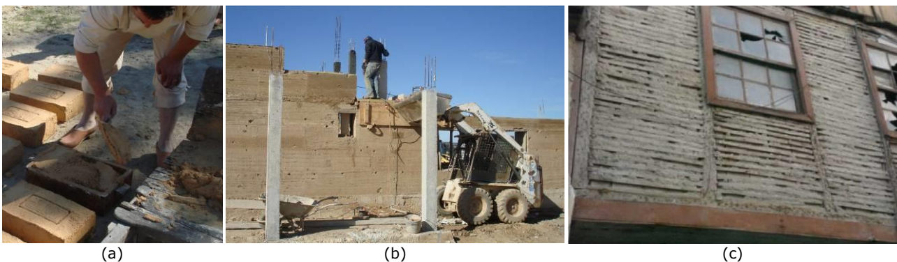
Figure 2 – Earth construction techniques: (a) adobes being manufactured; (b) construction of a rammed earth Wall; (c) external wall made of "tabique" (Pinto et al., 2010).
