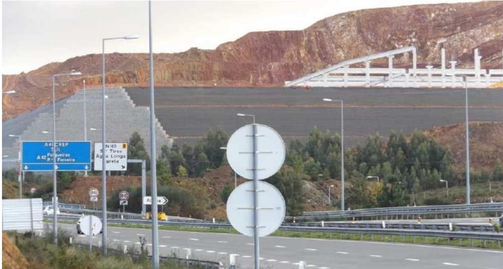
Fig. 2. Terra Link® Inferior Platform with Gabions facing system connection
