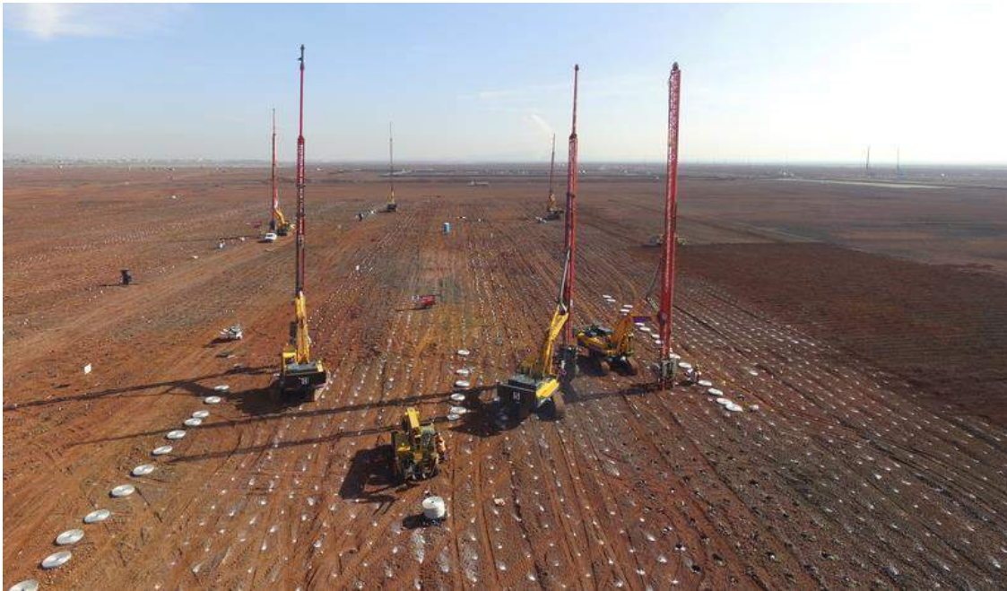
Figure 1. Execution of PVD below the future runways
