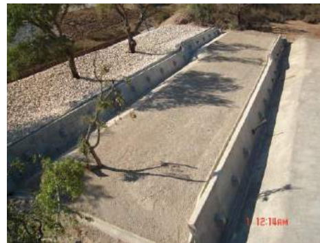
Photo 4. Permanent stabilization solution (2012)
