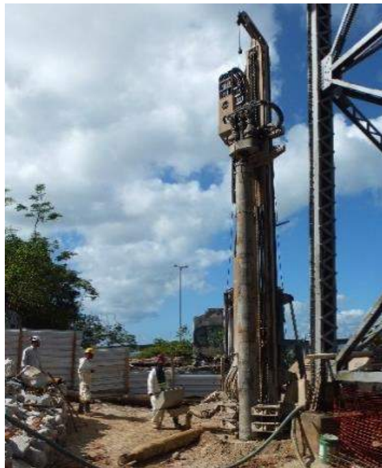
Figure 1. Execution of root-type piles
