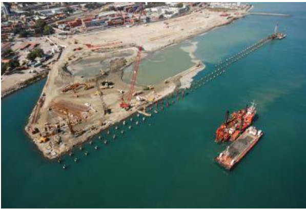
Figure 8: Sequence and stages of the embankment
