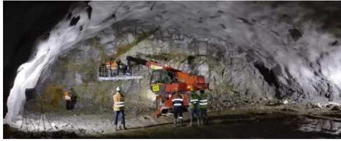
Figure 3. Excavation surface aspect (granitic rocky deposit).
