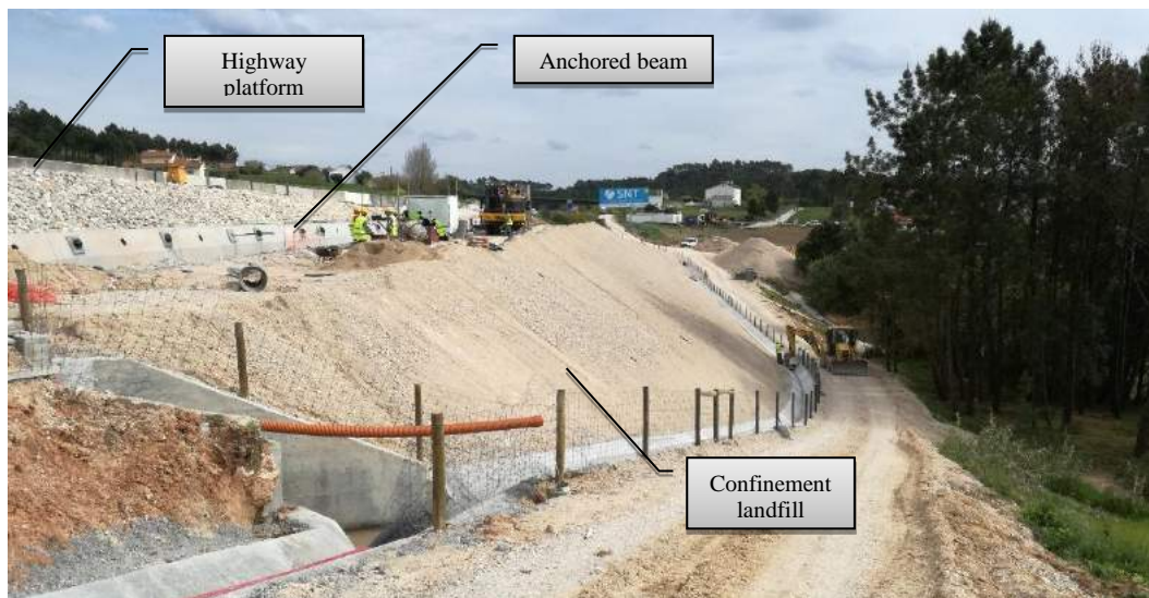
Figure 1. General view of the reinforcement and stabilization works.
