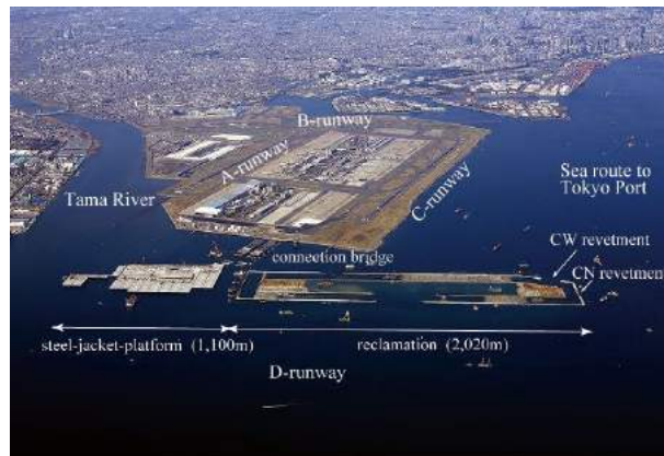
Figure 1. Sky view of construction site and existing airfield on March 15th, 2009 (by courtesy of the Tokyo/Haneda International Airport Construction Office).
