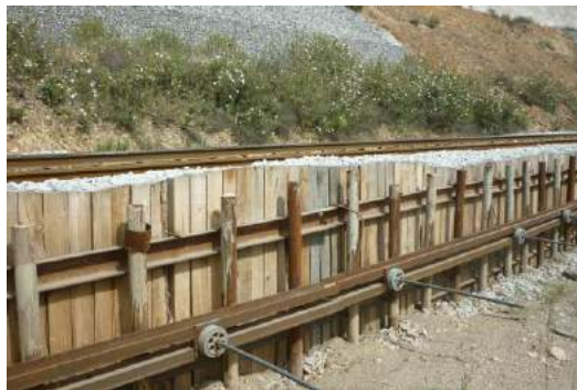
Photo 3. Temporary retaining solution (2011)
