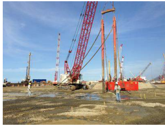
Figure 9: Execution of vibroflotation
