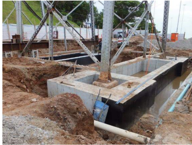
Figure 2. Execution of the blocks foundation
