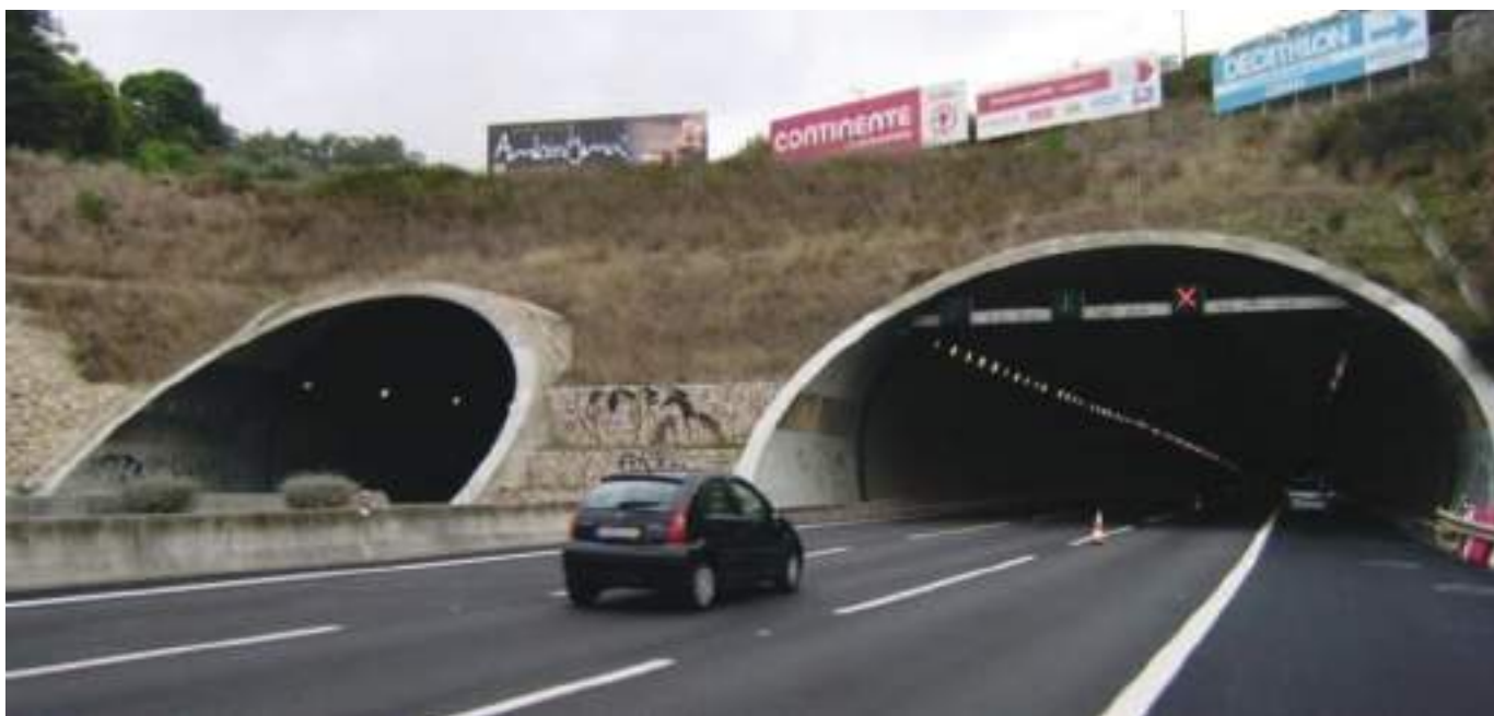
Fig. 01 Vista do emboquilhamento Sul-Poente (SW). View of the south-west portal.
