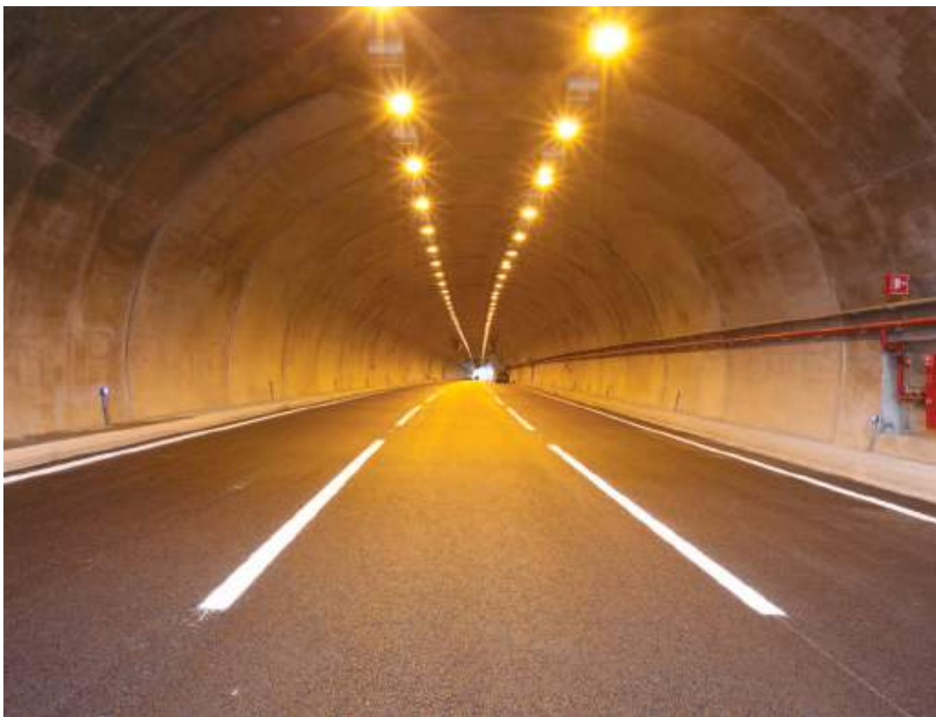
Fig. 01 Túnel do Covelo – A41. Covelo Tunnel – A41.
