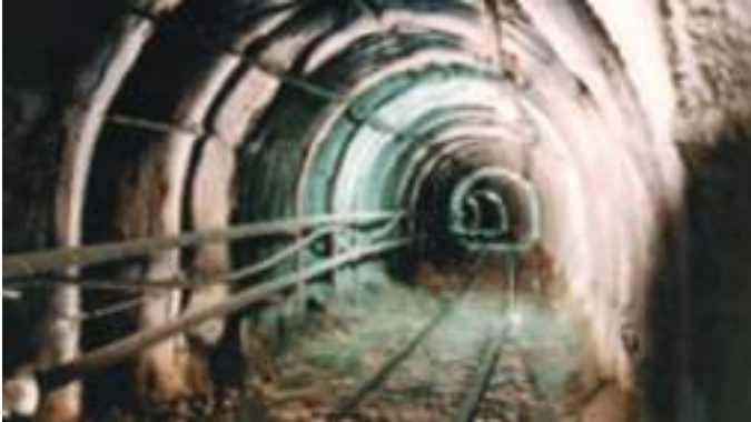
Interior da galeria do Túnel 2 Interior of Tunnel 2 gallery
