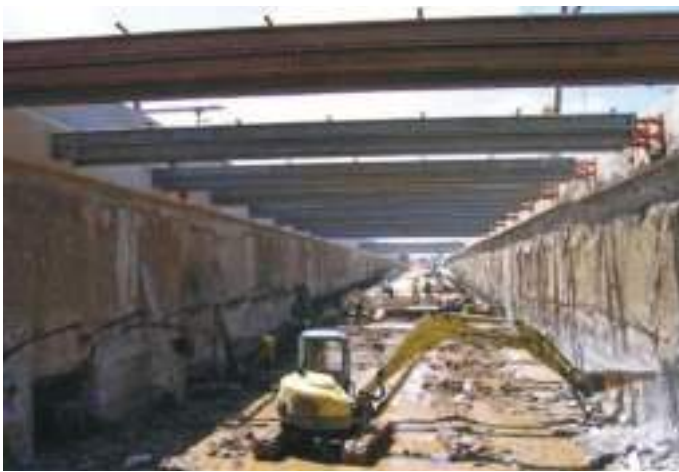
Execução dos recalces dos painéis e proteção com jet-grouting no tardo das paredes. Execution of re-injection of panels and protection with jet-grouting at the inside face of the walls.
