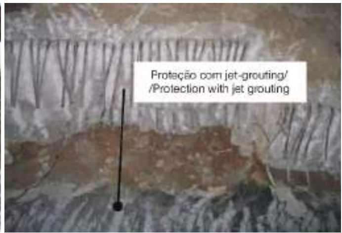
Execução dos recalces dos painéis e proteção com jet-grouting no tardo das paredes. Execution of re-injection of panels and protection with jet-grouting at the inside face of the walls.
