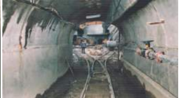
Interior da galeria do Túnel 1 Interior of Tunnel 1 gallery
