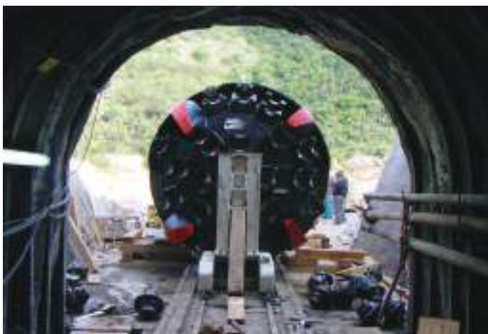
Fig. 03 Aspectos da tuneladora em montagem no emboquilhamento de jusante. Views of the TBM as it was being assembled at the downstream portal.
