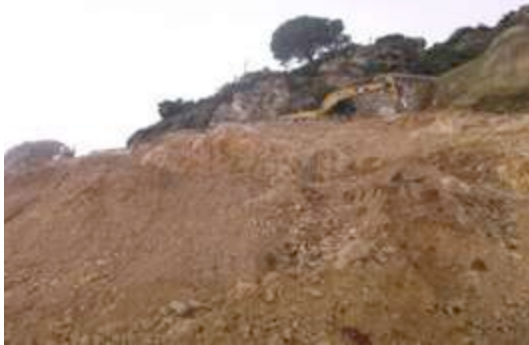
Figure 8. Limestone rock massif face at zone 2.3 (Nunes, 2015)
