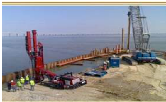
Figure 4. View of sheet pile driven operations from the site central area.
