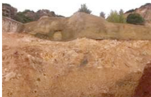
Figure 7. Limestone rock massif face at zone 2.2 (Nunes, 2015)
