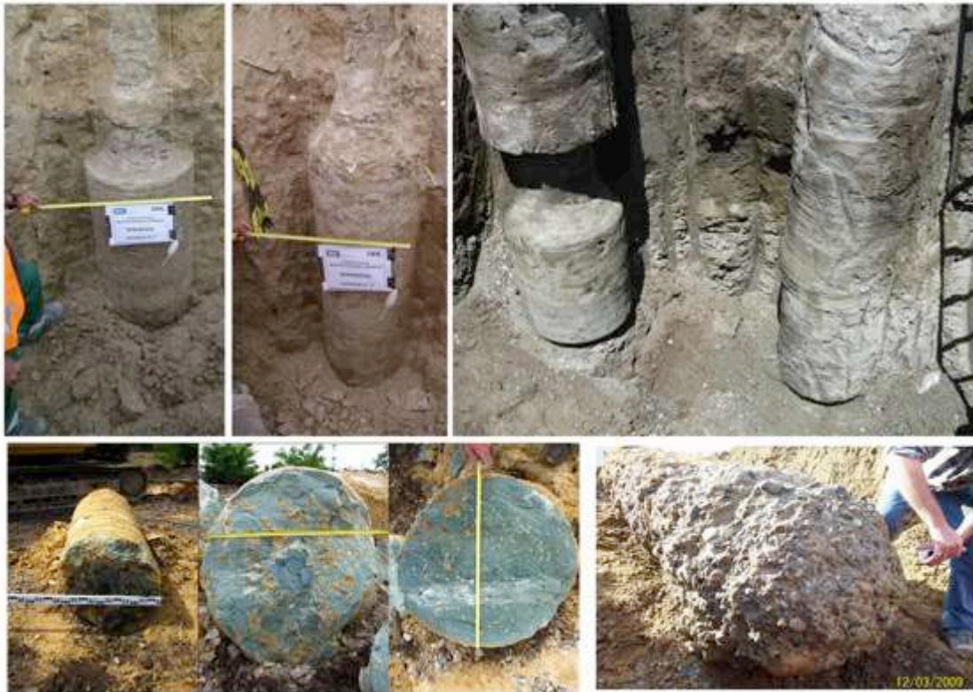
Figure 2. Springsol® columns executed in different soil types.
