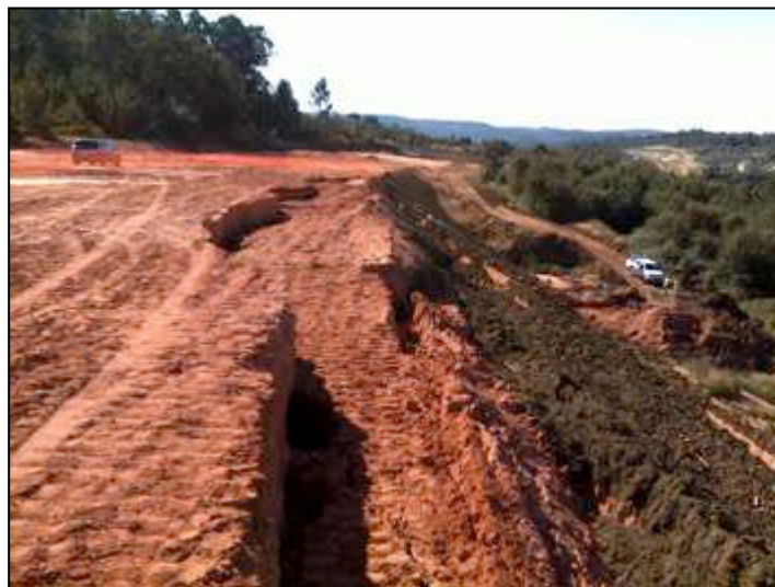
Figure 1. View of the sliding surface
