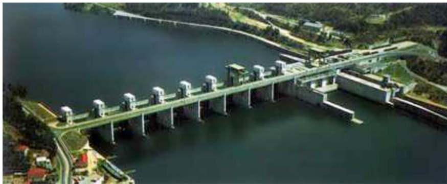
Figure 1. Crestuma-Lever dam aerial view.
