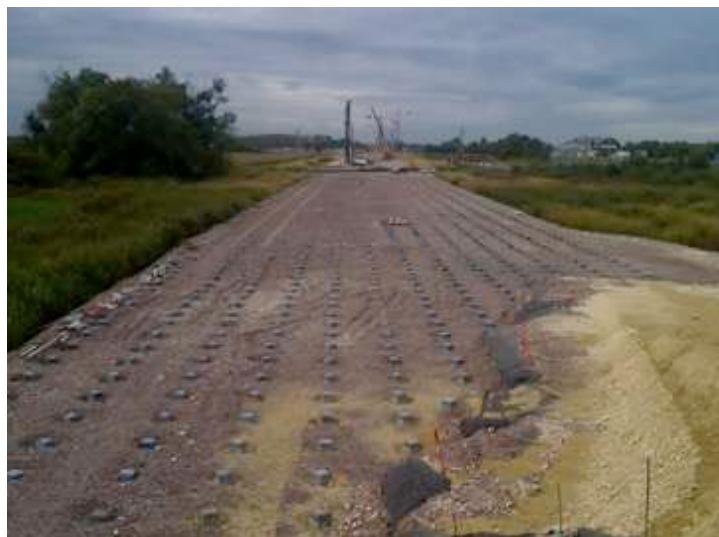
Figure 7. View of pile mesh from experimental embankment
