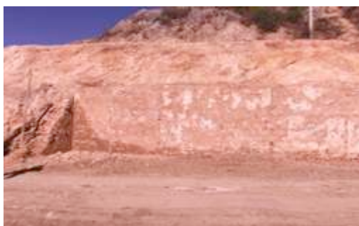
Figure 4. Limestone rock massif face at zone 2.1 (Nunes, 2015)
