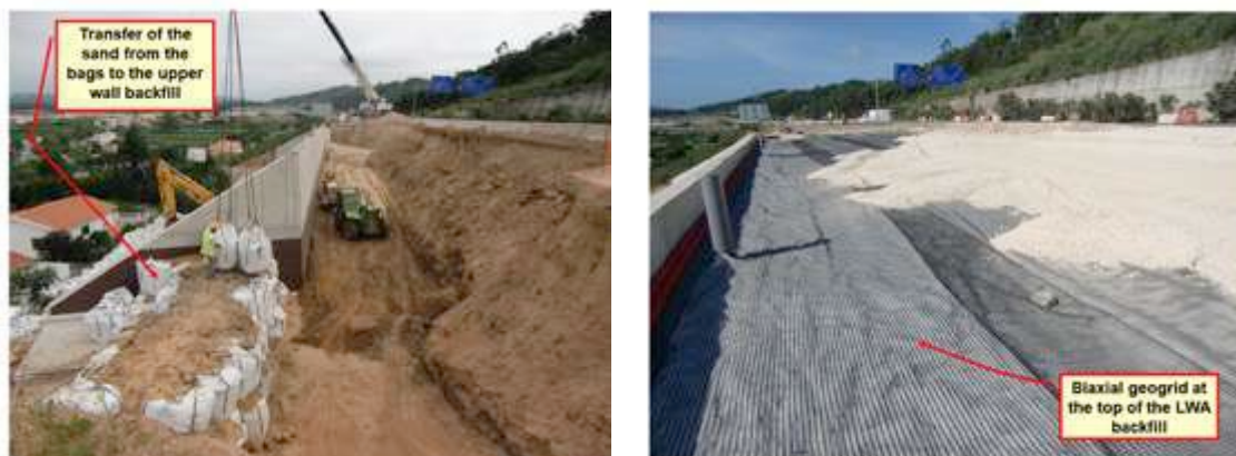
Figure 5. Views of the upper wall backfill works.
