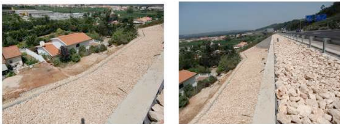
Figure 8. View of the finished stabilization works.
