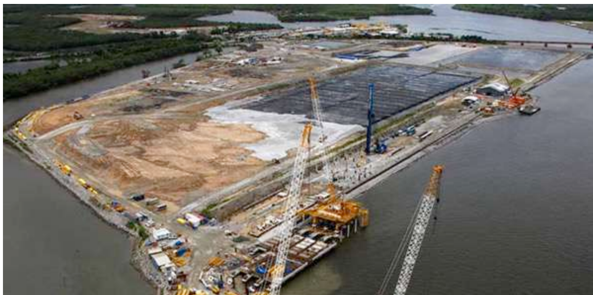
Figure 1. Geotube® dewatering of contaminated sediments
