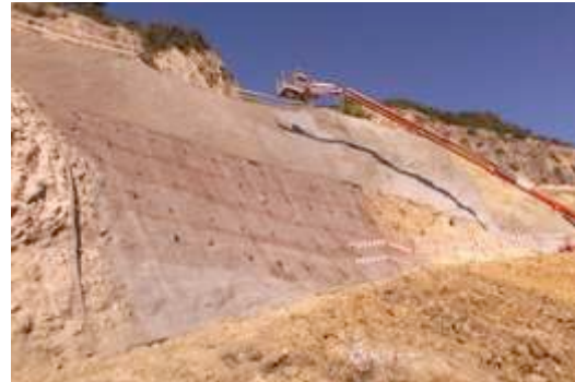
Figure 9. Limestone rock massif face at zone 2.3 (Nunes, 2015)
