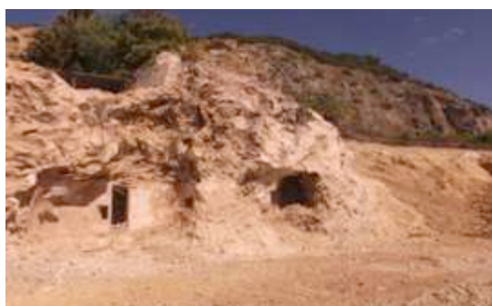
Figure 6. Limestone rock massif face at zone 2.2 (Nunes, 2015)
