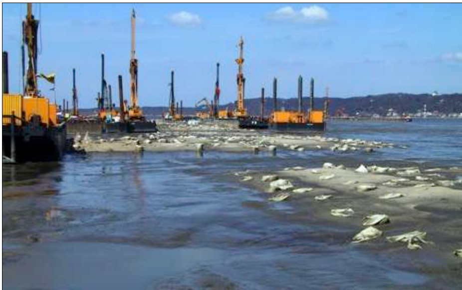
Figure 1. Installation of GECs (Ringtrac) over water and extremely soft mud
