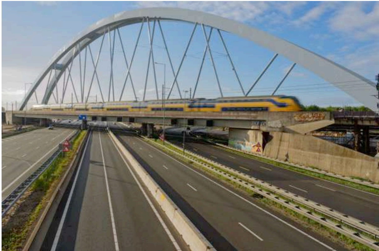
Figure 6: The bridge after placement on its temporary location with the old highway still in place ( http://www.nevesbu.nl )
