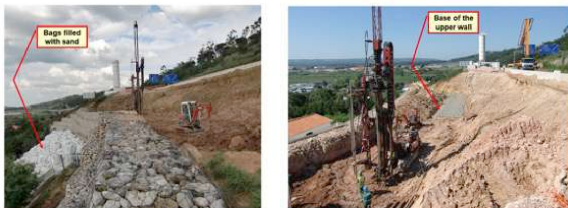
Figure 4. Views of the jet grouting works.
