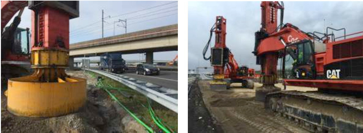
Figure 2. Compaction operations next and on stretches of the highway
