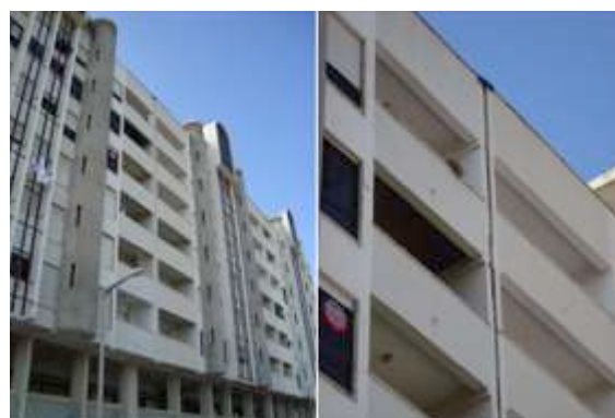
Figure 2. Deformations/Rotation of the affected buildings (Nunes, 2015)
