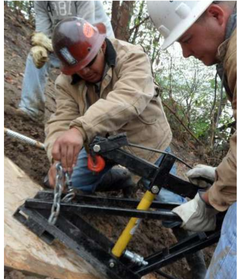
Anchor load testing and driving with percussion hammer
