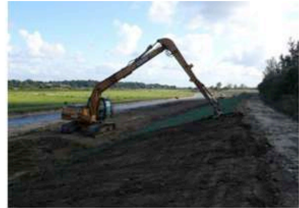
Embankment, Staffordshire, England
