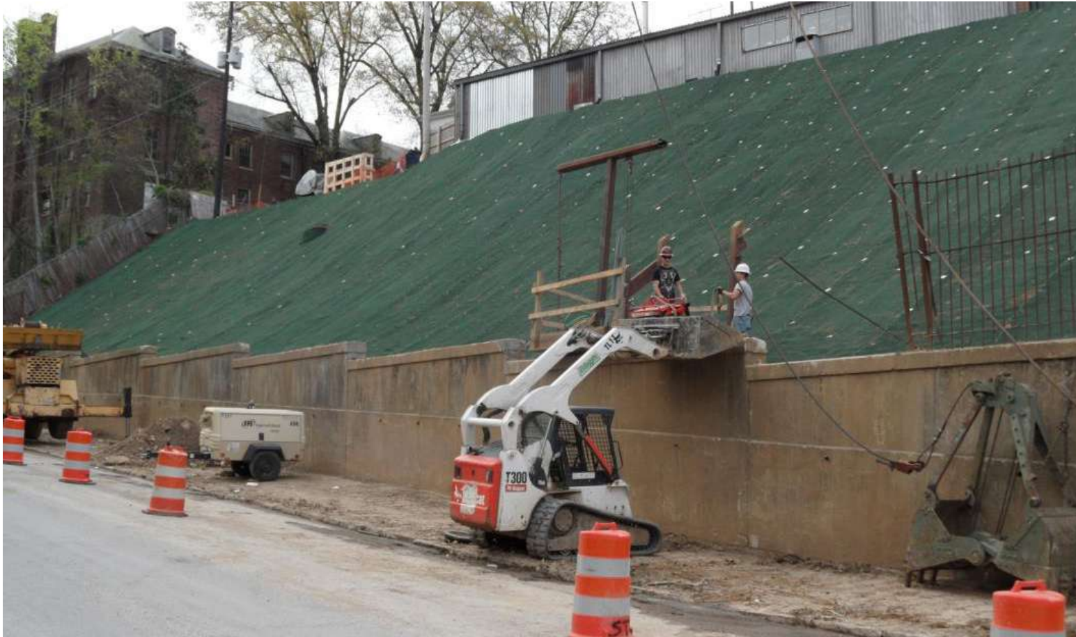
Small equipment used facilitating construction in limited easements
