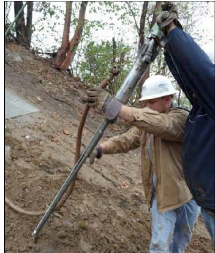
Anchor Driving with a Percussion Hammer
