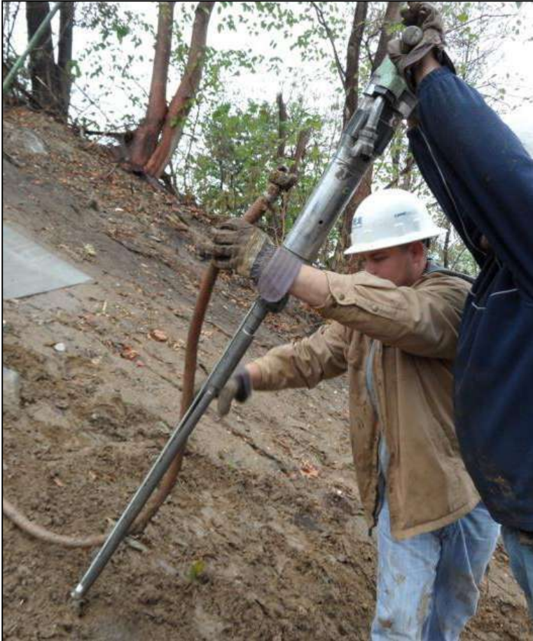
Anchor load testing and driving with percussion hammer
